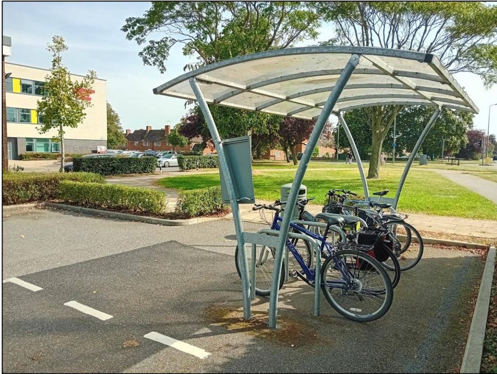
Figure 17: Covered Sheffield stands at Abingdon and Witney College, Abingdon
