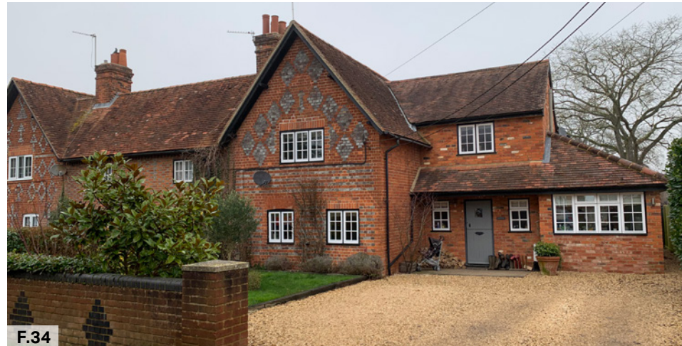
Figure 34: Local material used in a two- storey family house in Gravel Road Settlement, that demonstrates the incorporation of distinctive architectural elements on the facade as visual prompts for orientation and wayfinding
