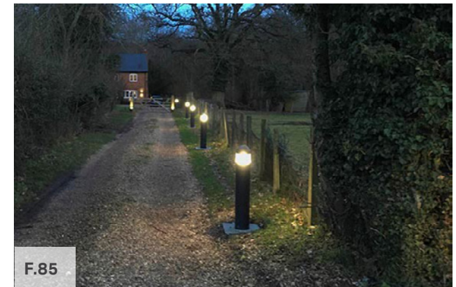
Figure 85: A negative example of exterior lighting on Common Lane, frequently left on throughout the night causing unnecessary light pollution. This is exacerbated by the design of the fittings themselves which reflect light upwards. In all cases PIR movement sensors should be fitted. (Source: Binfield Heath Parish Council)
