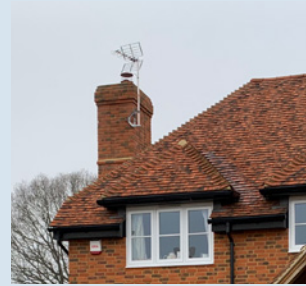
Plain tile and red brick chimney stack
