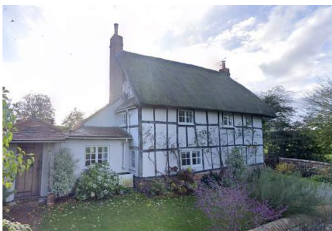
Figure 10: Frieze Cottage was originally part of the Crowsley Park estate, 18th Century Grade II Listed
