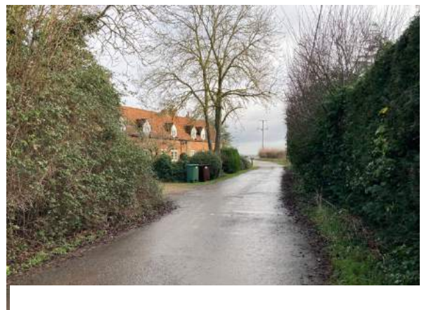
Figure 22: Typical 1.5 storey brick cottages
