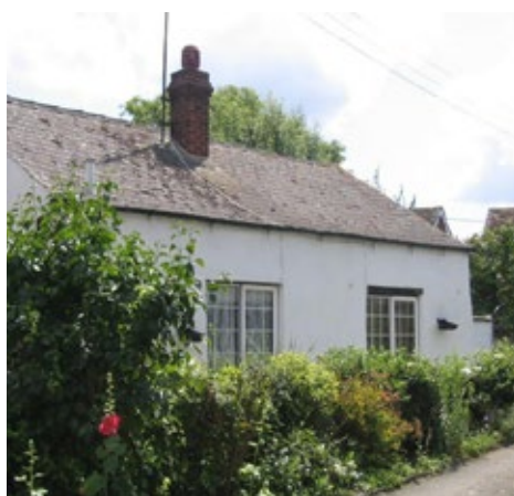
Former chapel at Bridge End
