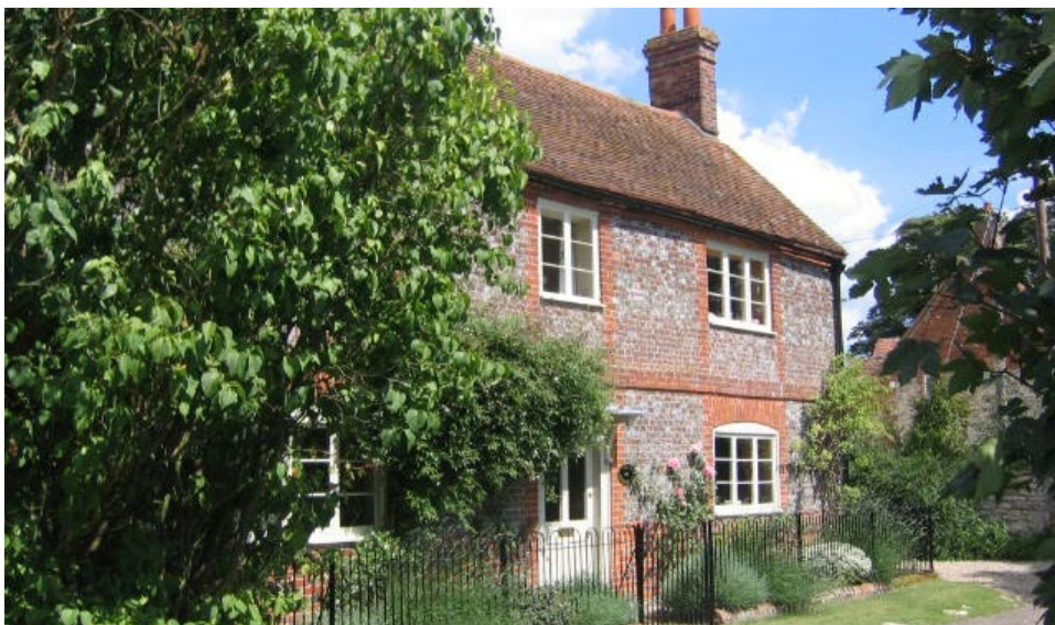
Overy Farm House
