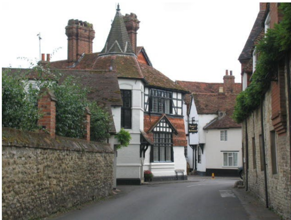
Rubble stone wall (above image, left) on Queen Street
