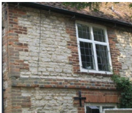
Clunch and brick at Lych Gate Cottage
