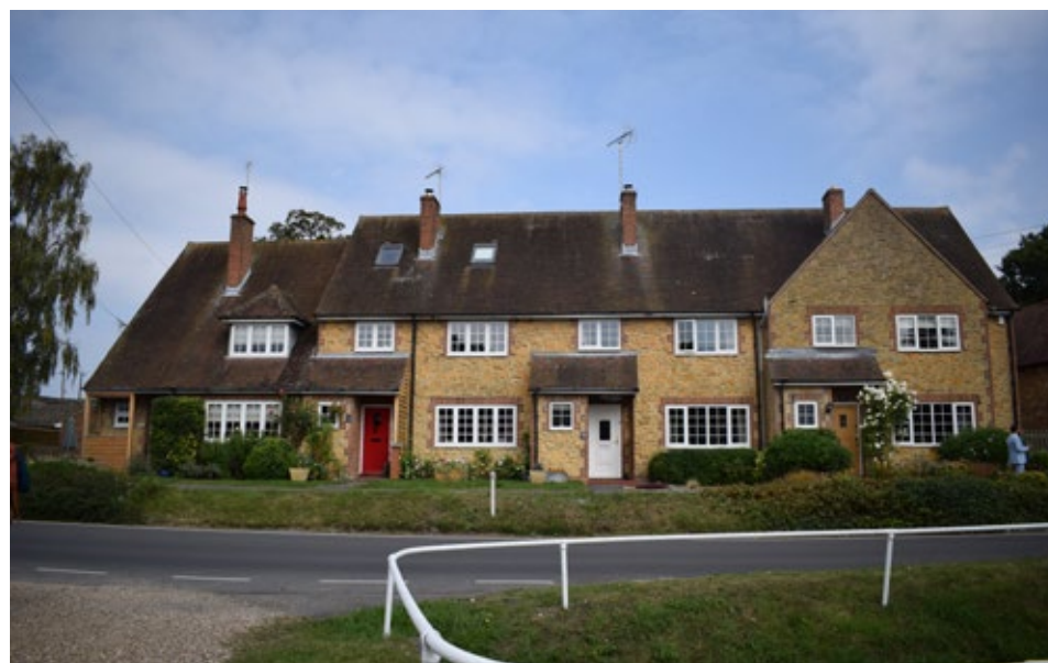
Fig 29. The Merton College Cottages (built 1976) are outside the CA but feature in the streetscape. An inappropriate iron-rich facing stone was used which has weathered to a dark yellow
