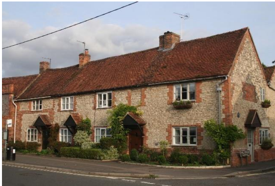
Chalkstone rubble with brick dressings
