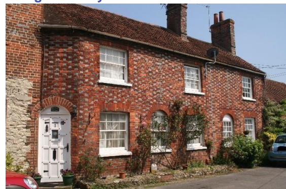
Chequer brickwork
