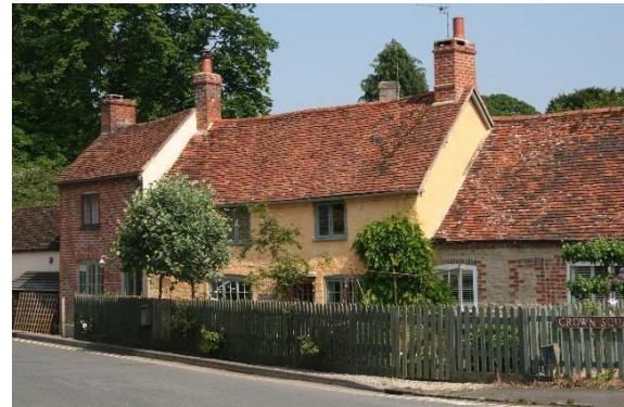
Lime-washed chalkstone rubble and orange/red clay tiles
