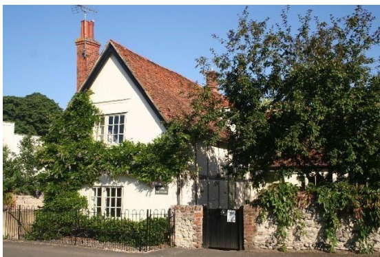
Timber frame with rendered masonry front
