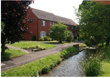
The Benson Brook at 46-54 Brook Street
