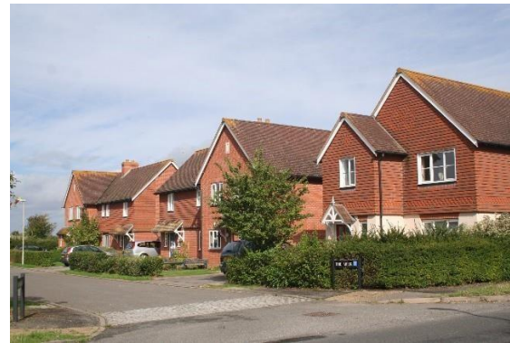
Steeper taller roofs at The Meer
