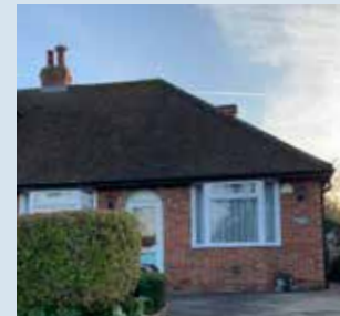
Hipped roof with tile
