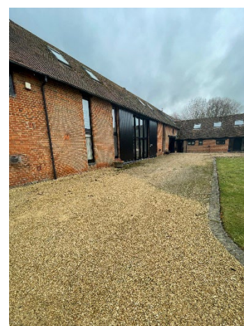
Manor Farm Development as an excellent example of the development of traditional farm buildings.
