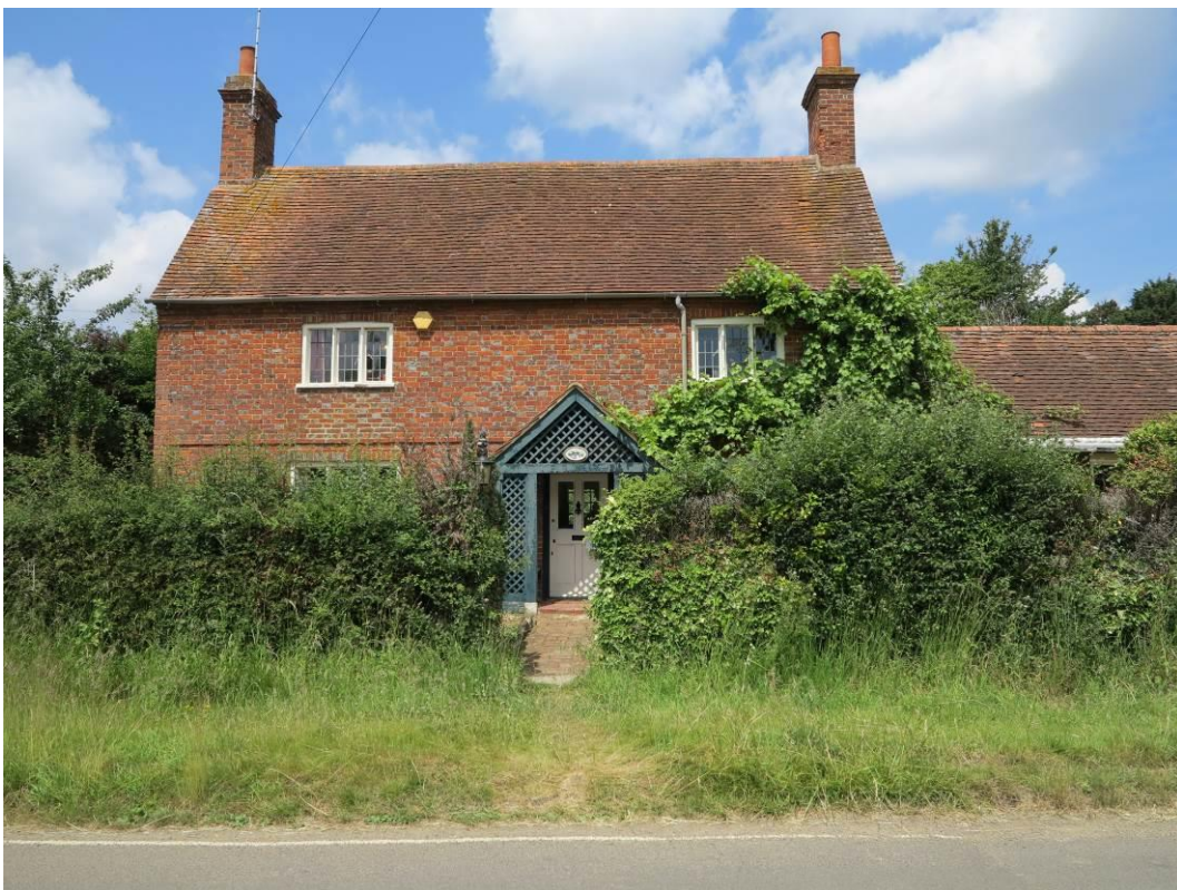
Plate 52: Vine Cottage, seen from High Street
