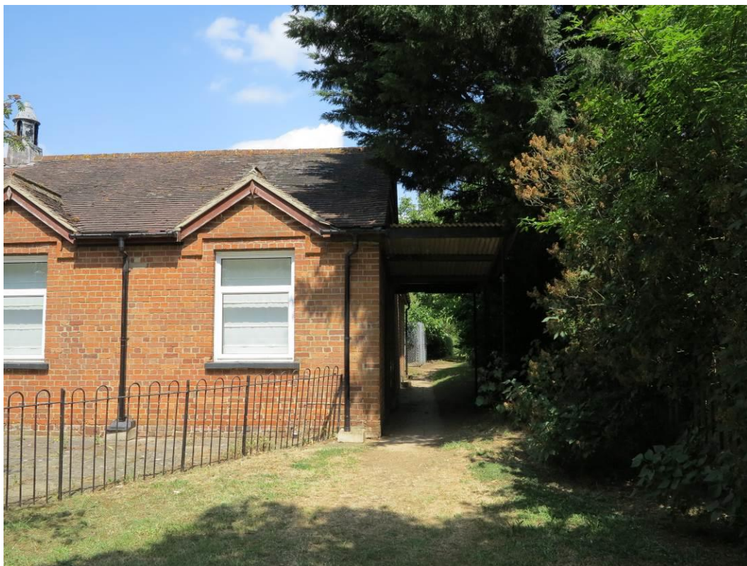
Plate 14: Entrance to eastern footpath, seen from Abingdon Road
