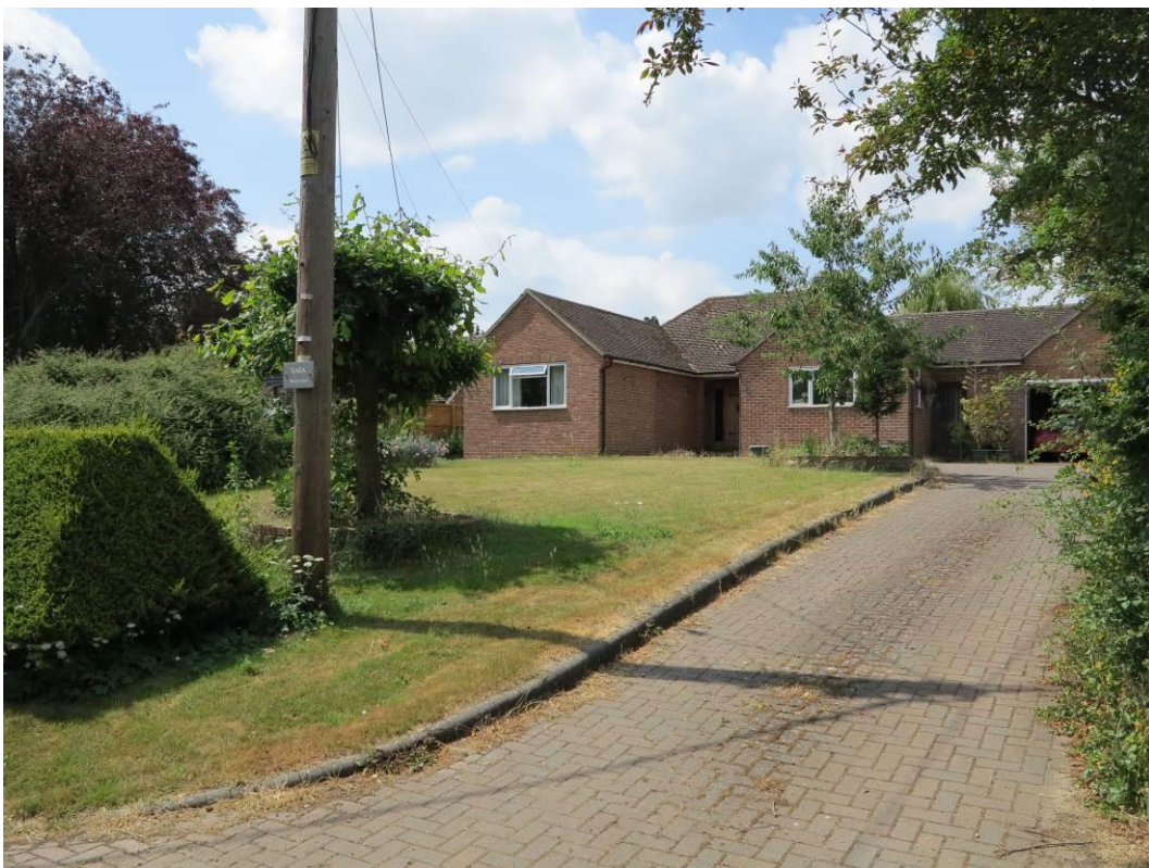
Plate 30: Typical 1960s/70s infill development on the western side of Watery Lane
