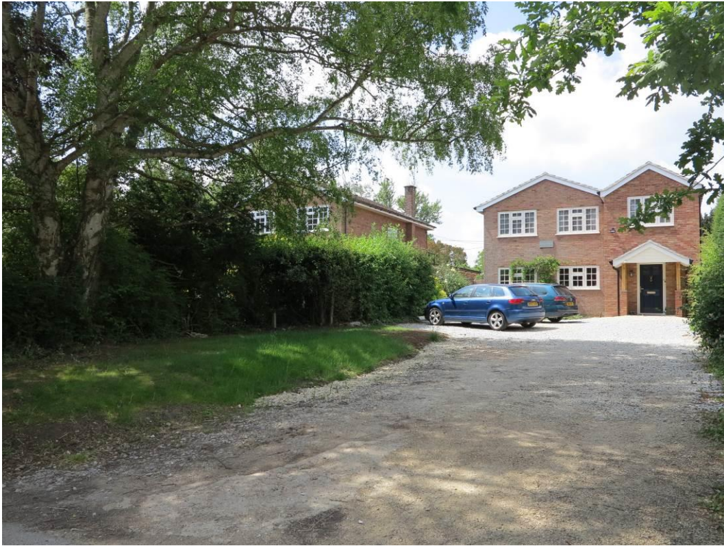
Plate 31: Typical 1960s/70s infill development on the western side of Watery Lane
