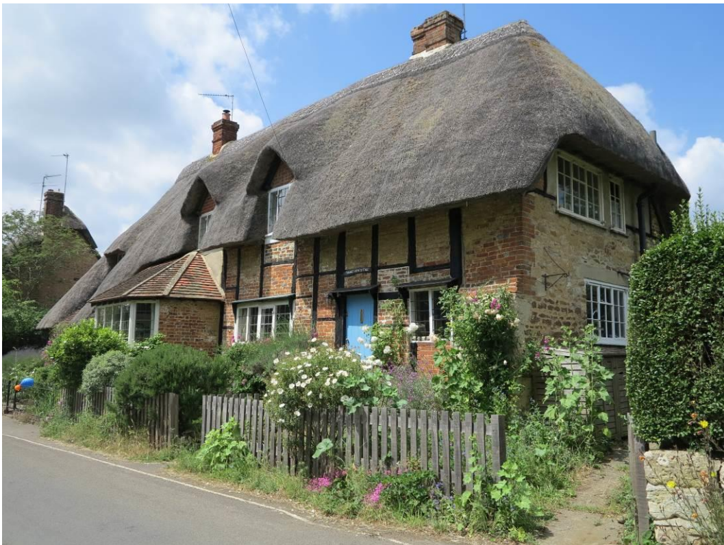
Plate 54: Clematis Cottage/Thames View
