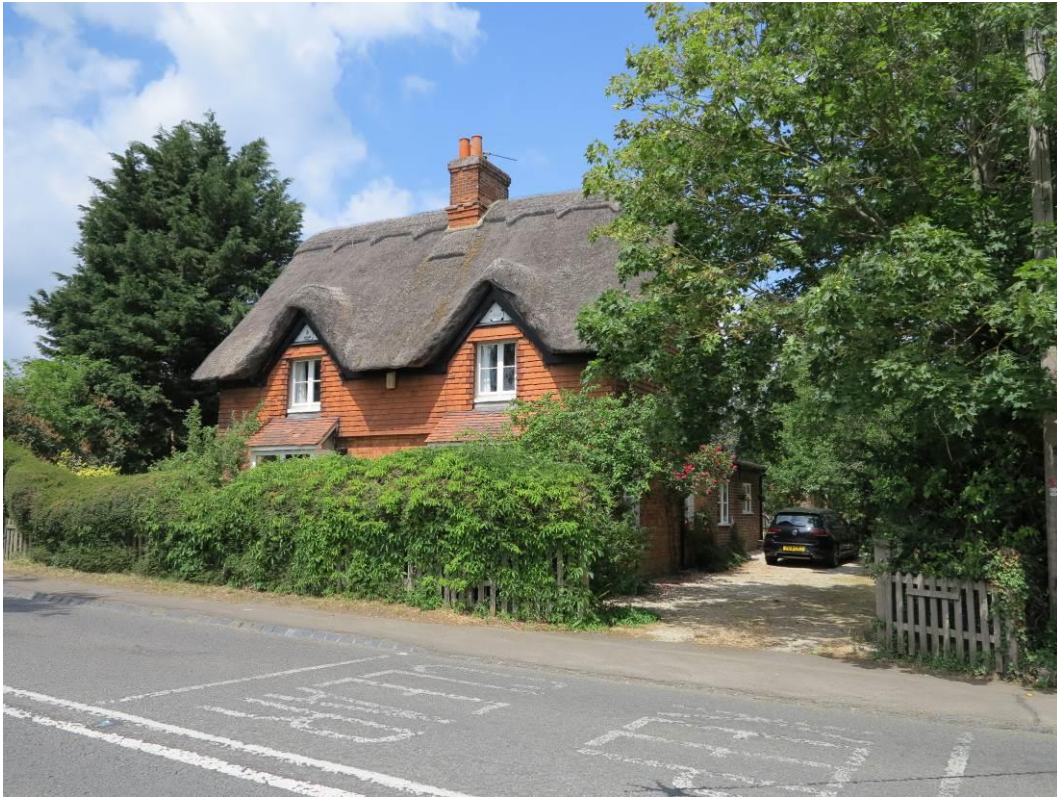
Plate 15: The Thatched House, seen from Abingdon Road
