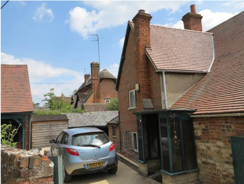
Plate 61: Looking from the footpath over the rear gardens of the houses fronting High Street between Vine Cottage and Clematis Cottage/Thames View
