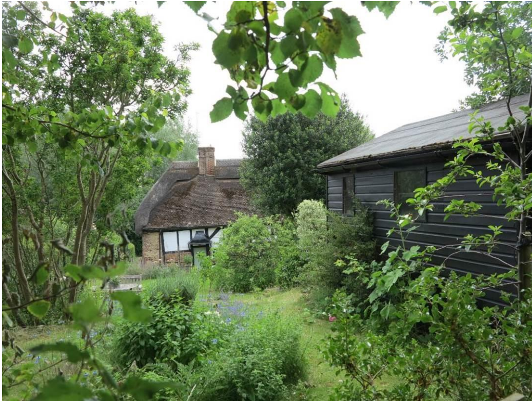
Plate 55: Looking from the footpath over the rear gardens of the houses fronting High Street between Vine Cottage and Clematis Cottage/Thames View
