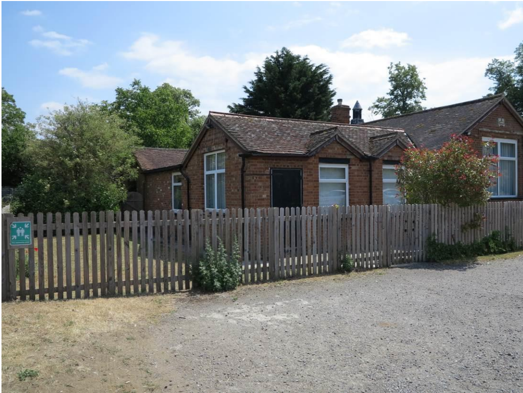
Plate 13: Village hall, viewed from car park
