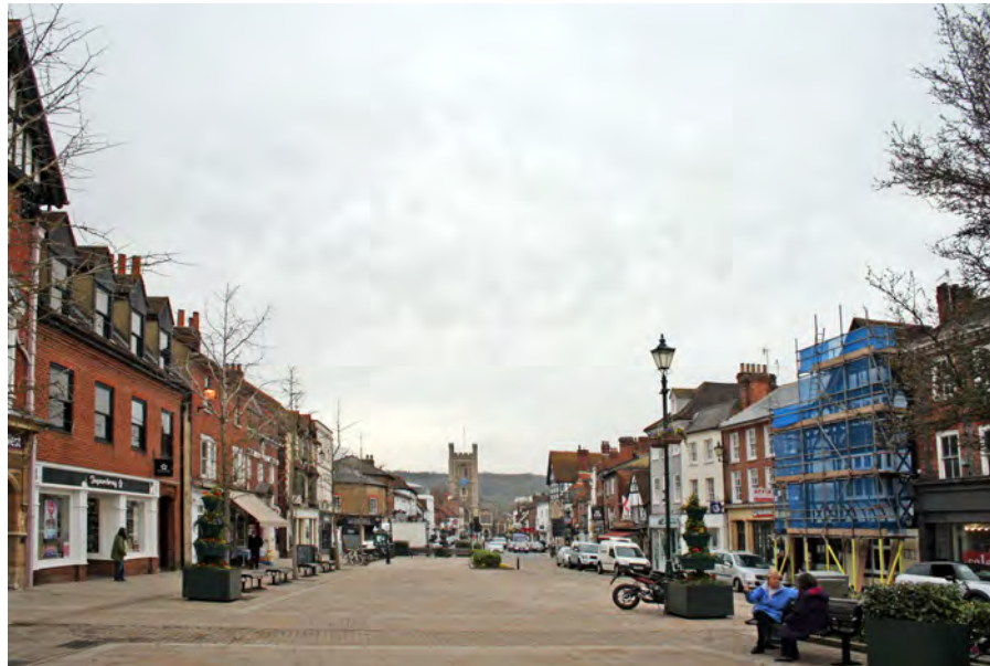
View of the Market Place showing its generous width and the landmark Town Hall
