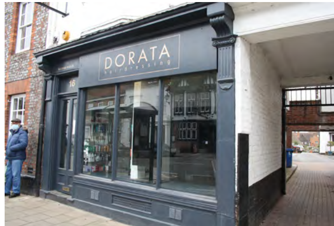
Historic shopfront on Hart Street
