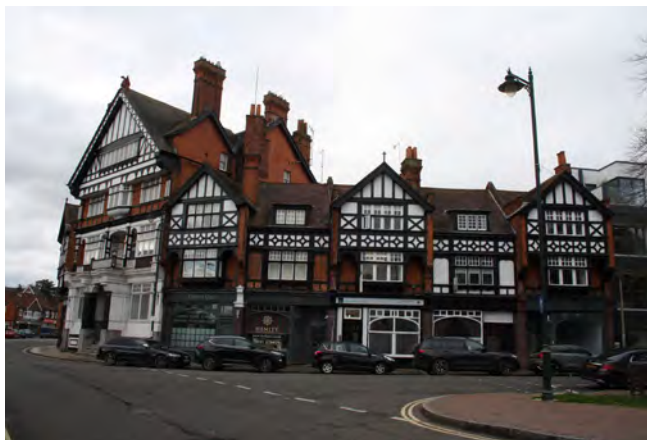
Imperial Hotel on Station Road characterised by deep gables, timber-framing and balconies
