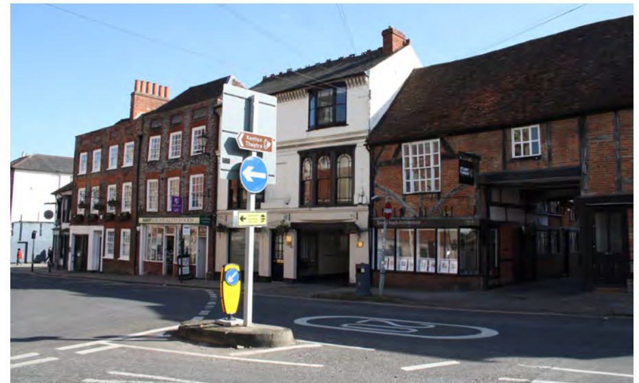
Commercial buildings at the lower (east) end of Gravel Hill
