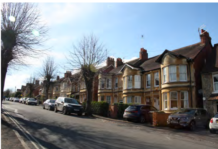
St Andrew's Road, showing the generous detached and semi-detached dwellings
