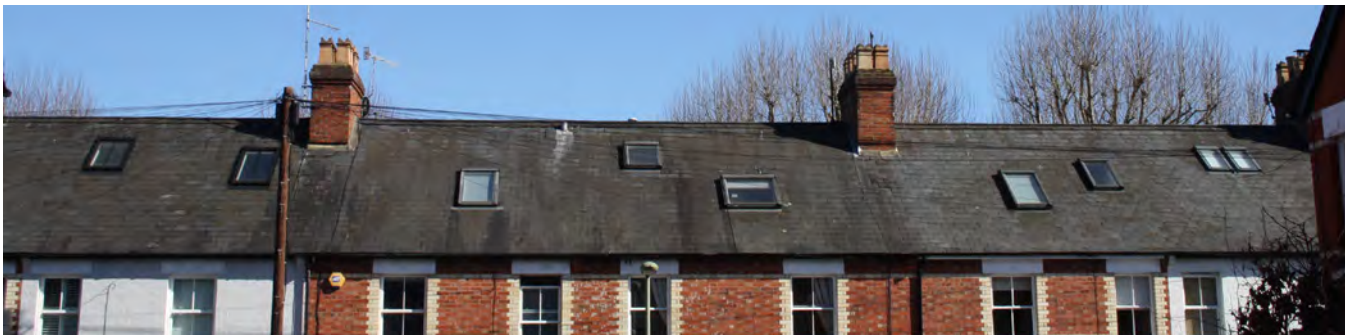
Skylight windows to front elevations
