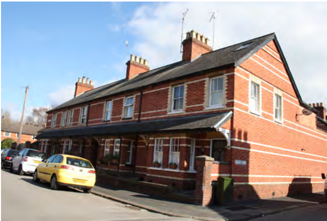
A terrace on Park Road showing verandas with fish scale tiles and low brick wall and gate pier boundary treatments.
