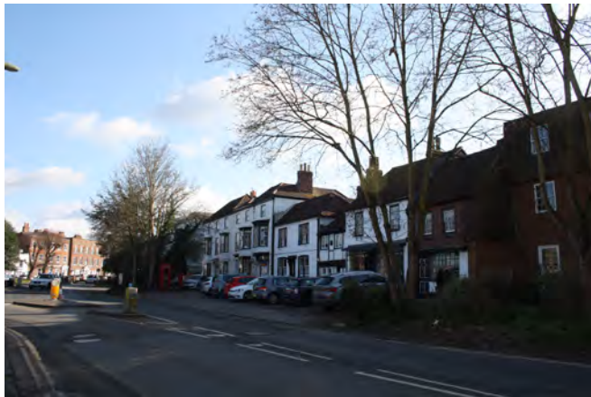
Dwellings and retail units at the south-west end of Northfield End
