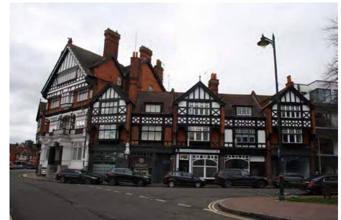
The largescale Imperial Hotel and associated buildings
