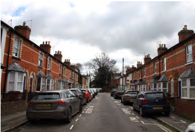
Small scale terraces on Albert Road
