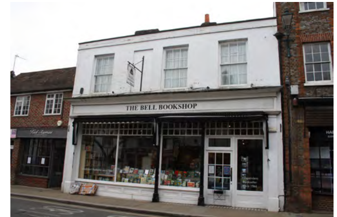
Historic shopfront on Bell Street
