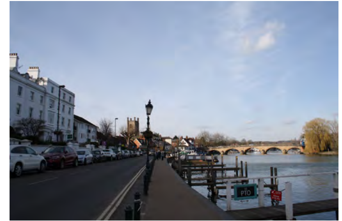
View along Thameside towards Henley Bridge and St Mary's Church
