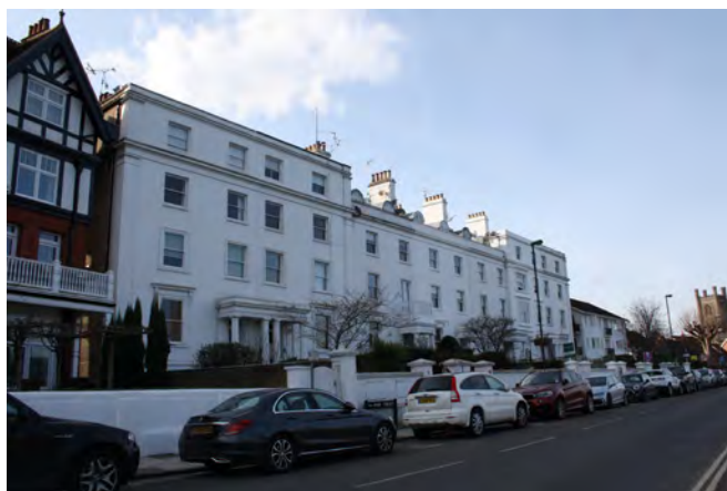
Four-storey River Terrace at the south end of Thameside
