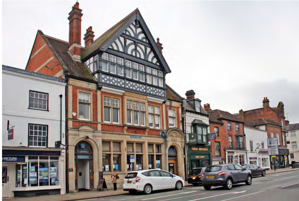
Stone and timber-frame detailing to a bank on Hart Street
