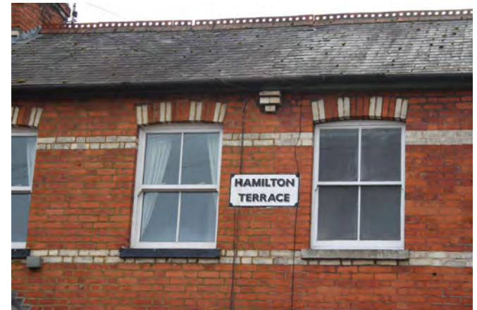
Detail of terrace with decorative brick banding and name plaque
