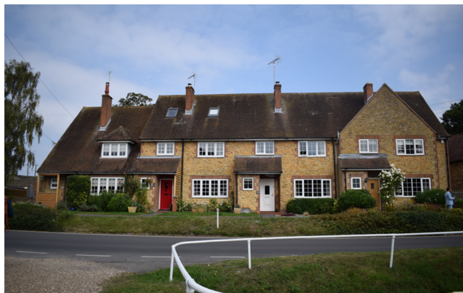
Fig 28. The Merton College Cottages (built 1976) are outside the CA but feature in the streetscape. An inappropriate iron-rich facing stone was used which has weathered to a dark yellow.
