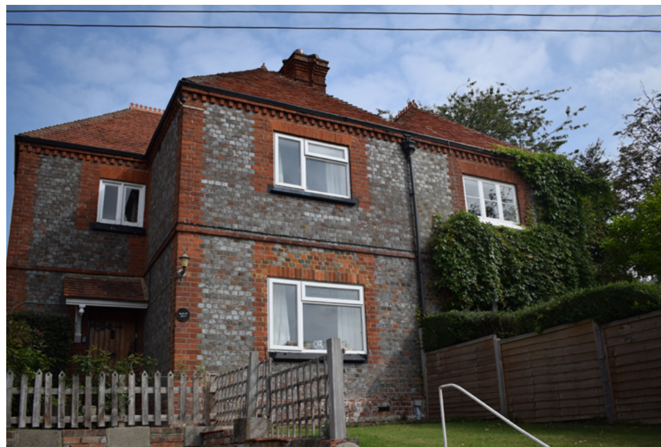
Fig 27. Dharwar Villa, which has had its original casement windows replaced.
