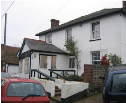
Fig. 26. Former village shop and post office
