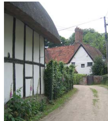
Fig. 30. The Priory and Old Priory Cottage on Little Lane
