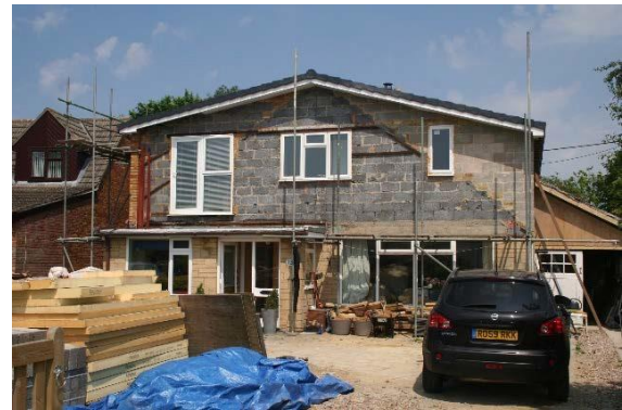
Bungalow modification underway at St Helen's Crescent
