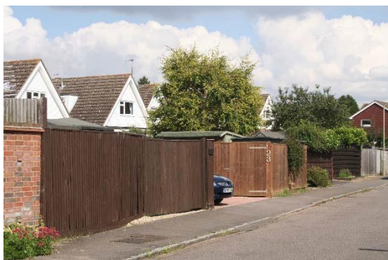
The "rear" aspect of chalets at St Helen Way
