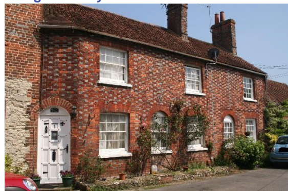
Chequer brickwork
