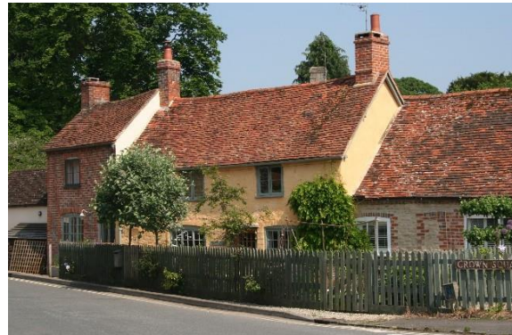
Lime-washed chalkstone rubble and orange/red clay tiles
