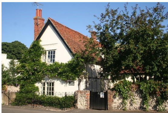
Timber frame with rendered masonry front
