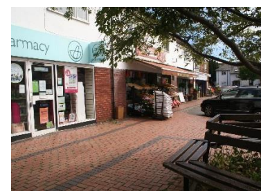
Paving scheme in front of the parade
