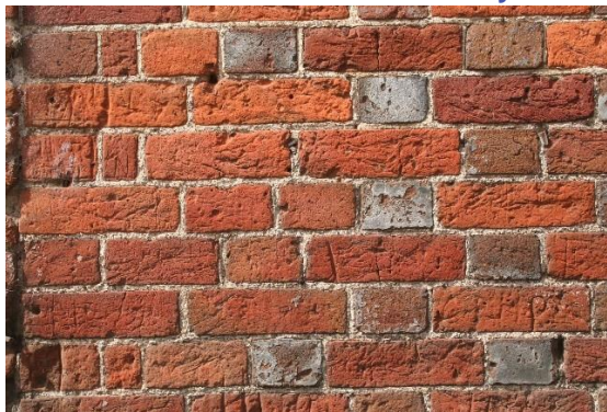
Orange/red brick with vitrified blue/grey headers
