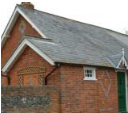
Fig 1. Diaper patterning in brickwork using burnt headers
