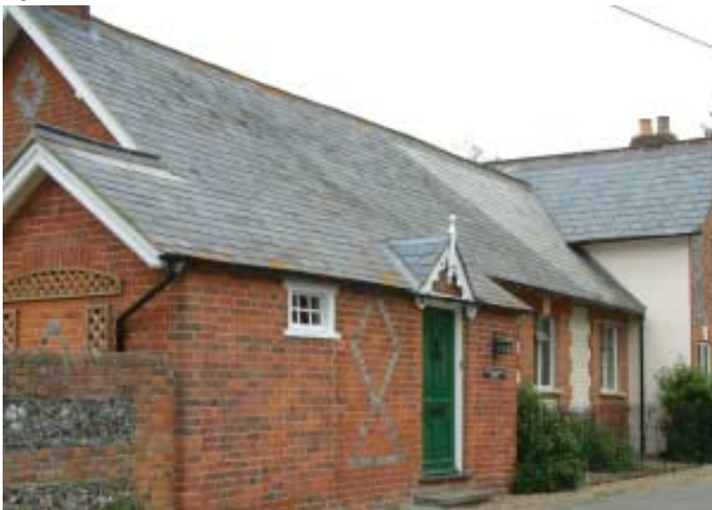
Fig 13. The Old School House
