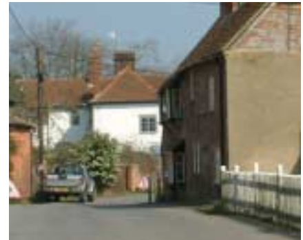
Fig 9. Close knit buildings on Thorpe Street
