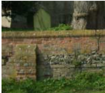
Fig 3. Brickwork at St. Michaels Church
