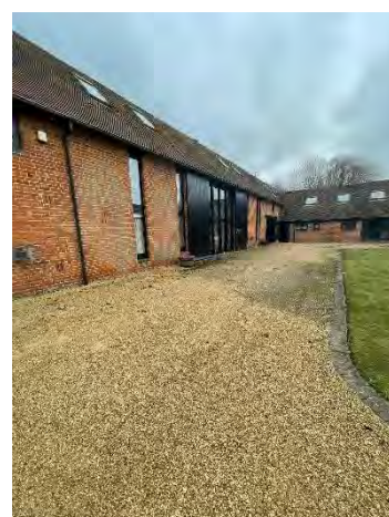
Manor Farm Development as an excellent example of the development of traditional farm buildings.
