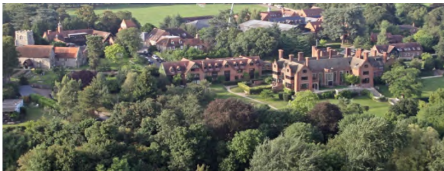
Figure 49: Aerial view of the College and Church
