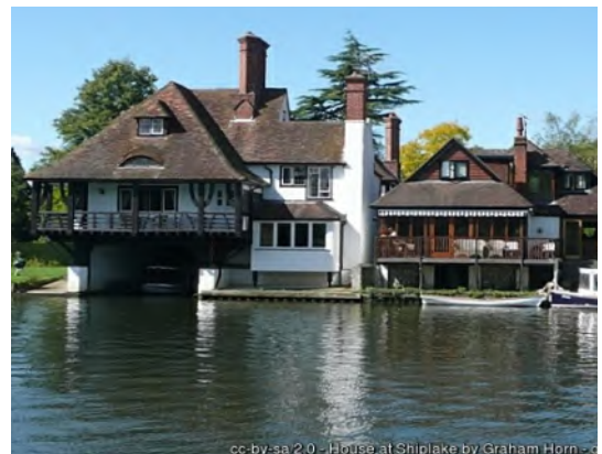
Figure 70a: Houses are built on the waters edge elevated to take into account flood waters and allow for integrated boathouses
