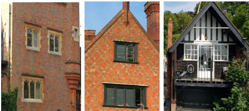
Figure 55: Detailing, fenestration, and materials including detail brick diaperwork on college buildings with low key materials found on the boathouse
