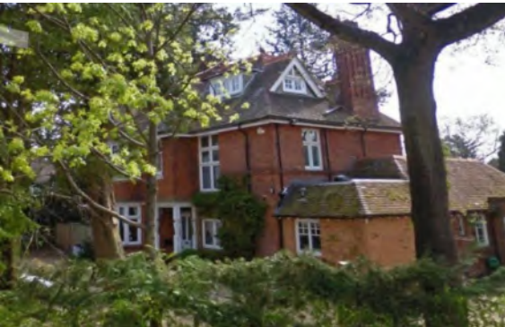
Figure 75: Red brick with plain clay tile and timber detailing, windows and doors predominate
