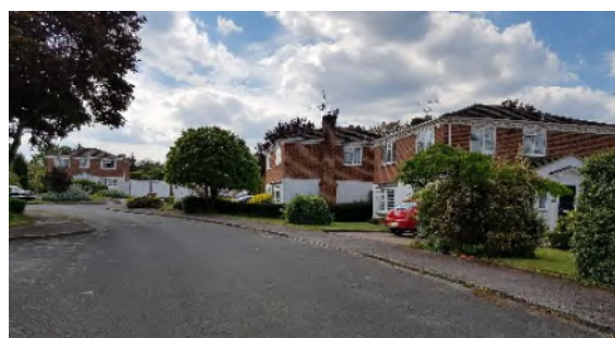
Figure 88: Housing in Brocks Way - detached or link detached set in open plan gardens.
