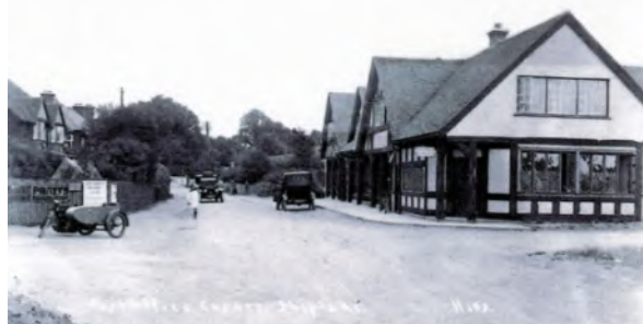
Figure 5: Lower Shiplake Corner Store (now demolished)
