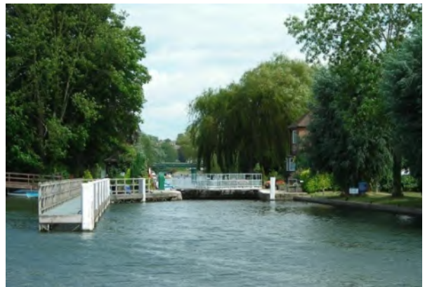
Figure 106: The view of the Lock looking down the Thames. The view is framed by mature tree planting and the Lock Keepers cottage.
