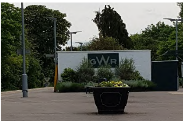
Figure 37: The former station buildings and the station modernised
