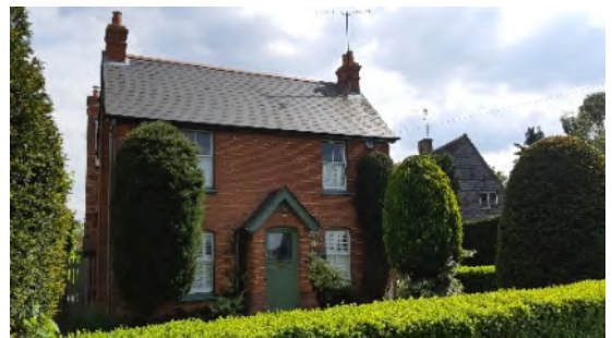
Figure 93: The retention of original features is essential in retaining character such as at Newlands, above
