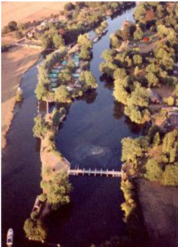
Figure 112: Aerial view of Shiplake Island with the lock beyond
