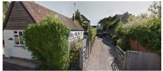
Figure 91: some of the older houses on Orchard Close, Shiplake. Old Bell House (in distance) (formerly Old Bell Cottage and Ballabeg [left] served the former Orchard on this site. Properties benefit from views over fields.
