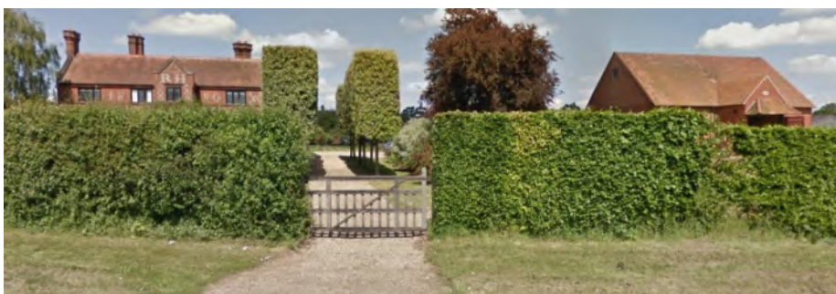
Figure 16: Siplake Farm House and Buildings
