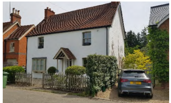
Figure 92: Older Victorian cottages need sensitive restoration such as the above example at Walnut Tree House
