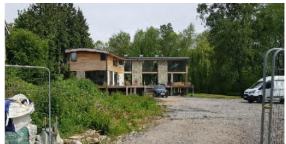
Figure 67: Replacement dwelling under construction
