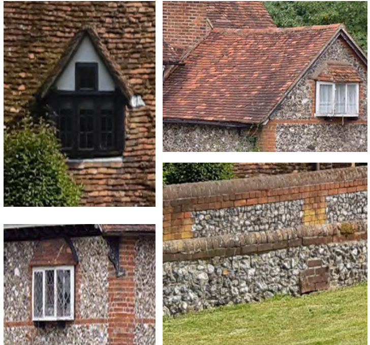
Figure 54: Detailing, fenestration, wall and roof coverings - highlighting brick and flint walls, play clay roof tiles and individual detailed window treatments
