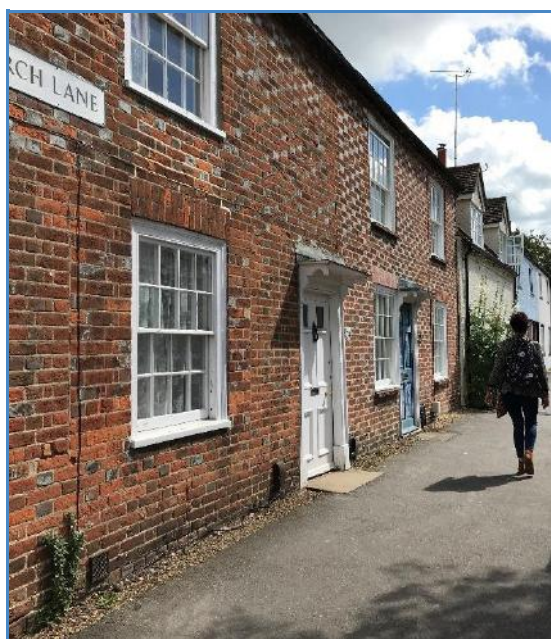
C18 vitrified header brickwork, Church Lane
