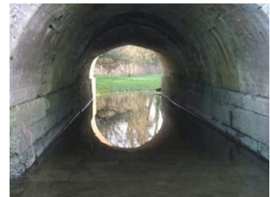
Figure 2.1 Wheatley Bridge, the remaining pointed arch of the medieval bridge can still be seen inside the reconstruction of 1809
