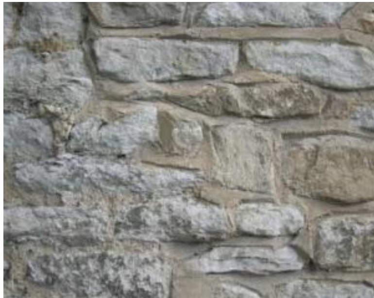
Original lime mortar and later cement repointing
