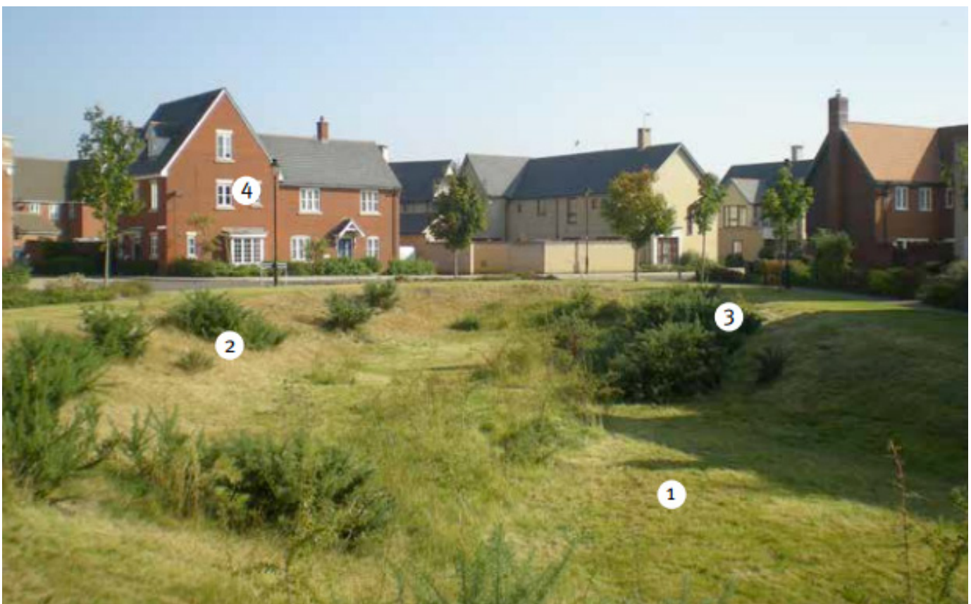
Infiltration basin at Ravenswood
