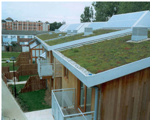
Example of an extensive green roof (Maidenhead)
